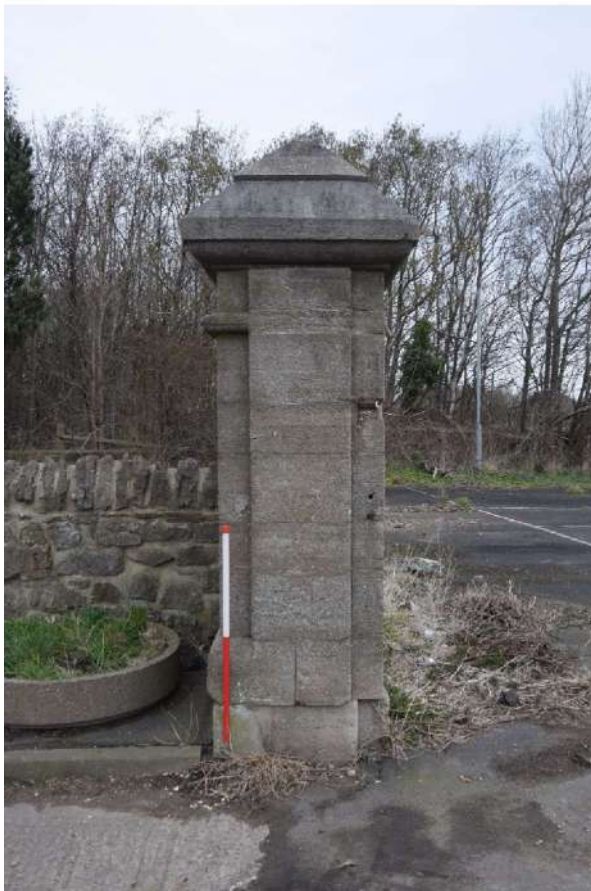
Photo 42: North pier of Whitburn Colliery, looking north
