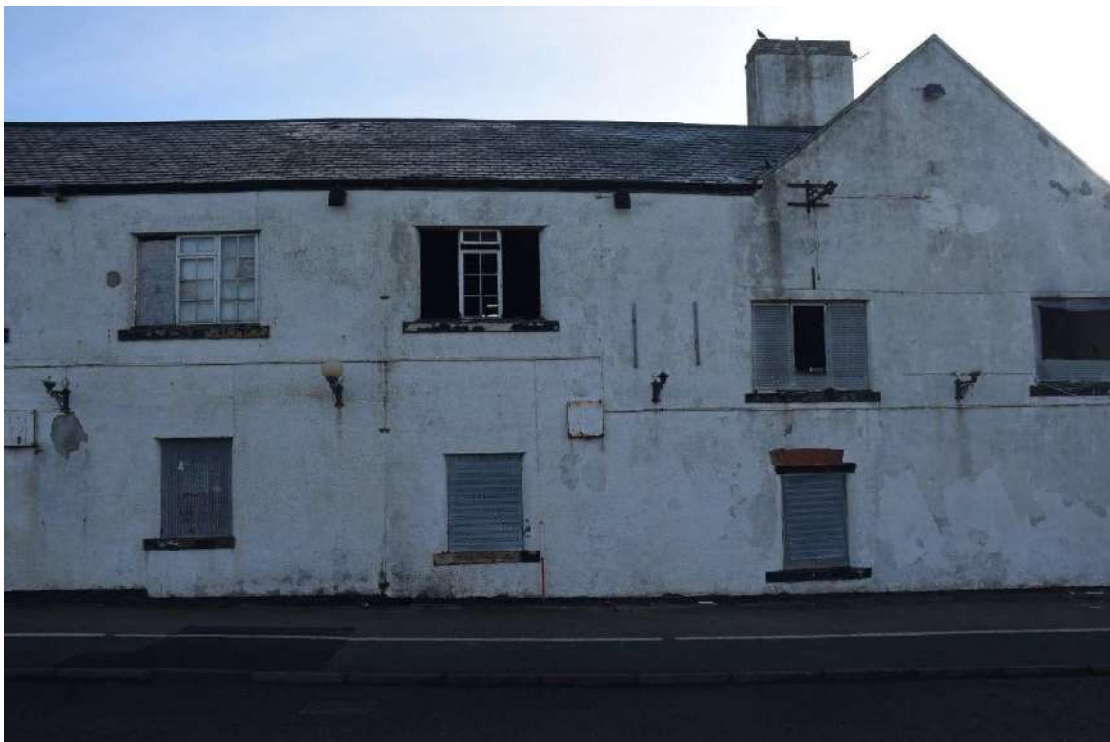
Photo 14: West-facing elevation of the south end of the west range, looking east
