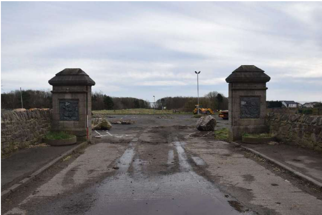
Photo 40: Gate piers forming the original entrance to Whitburn Colliery, looking east
