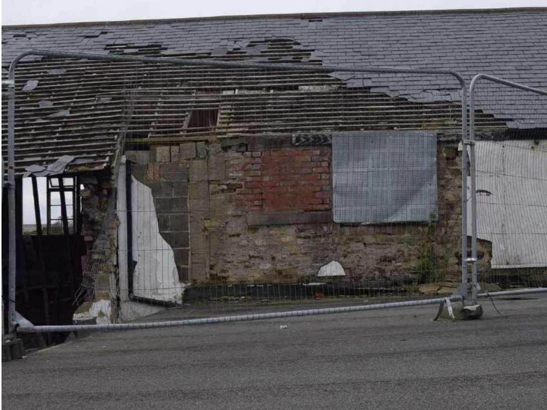
Photo 19: East-facing elevation of the west range showing the quoins of the southernmost cottage and a blocked window, looking west
