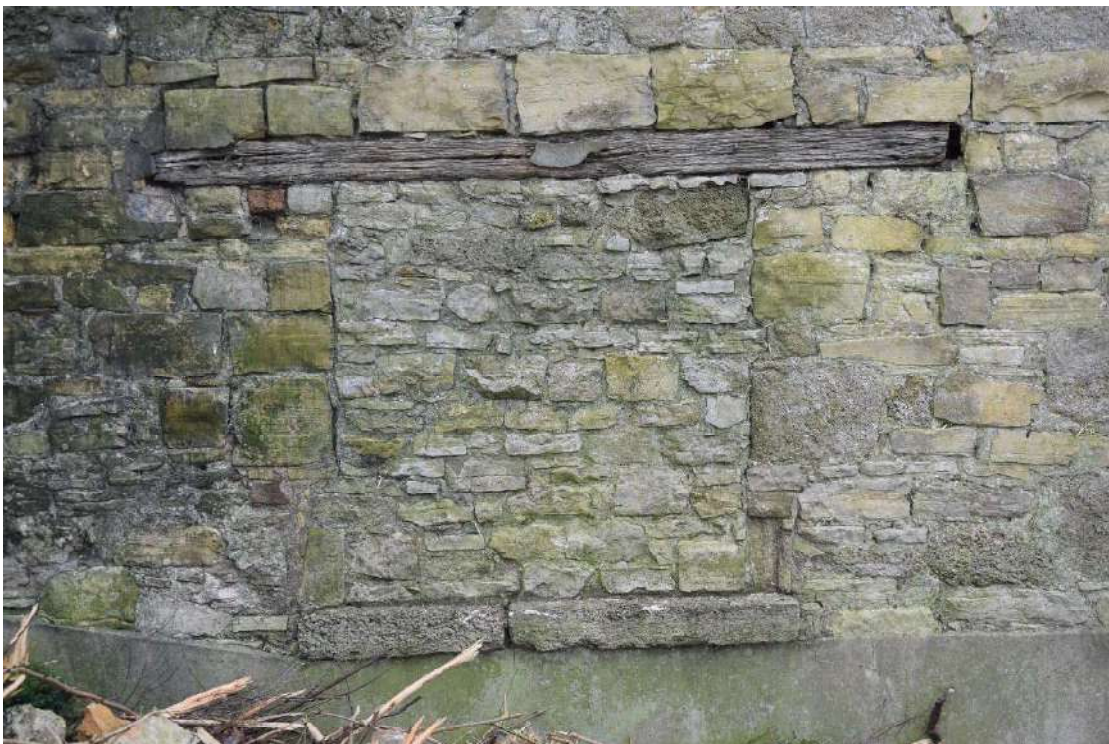
Photo 30 (below): Blocked window in the south face of the ground floor of the eastern extension, looking north
