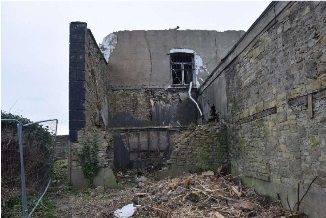
Photo 35: East gable end of Hope House, looking west
