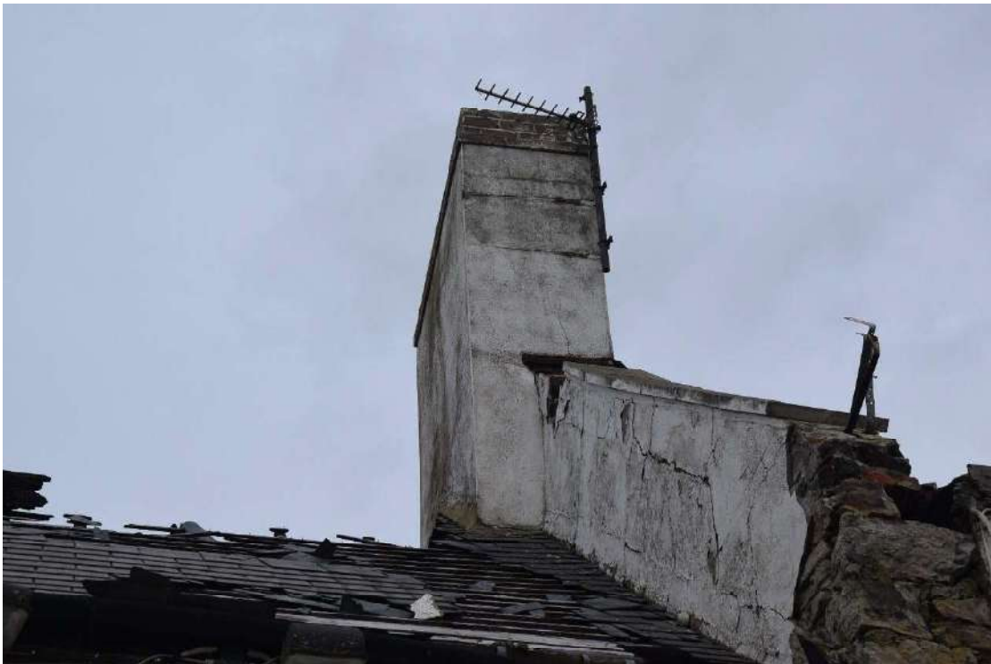
Photo 4: Western chimney of Hope House, looking north
