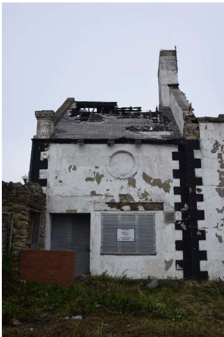
Photo 5 (left): Western extension to Hope House, looking north
