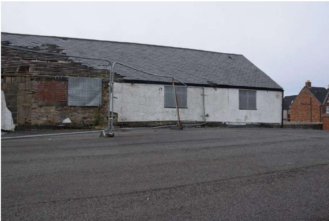
Photo 20: North end of the east-facing elevation of the west range, looking north-west
