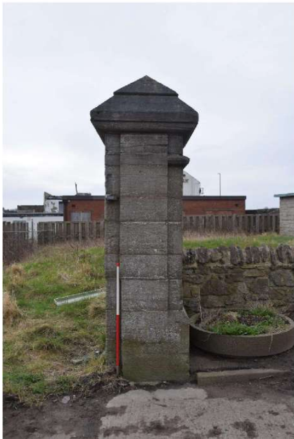
Photo 46: South pier of Whitburn Colliery, looking south
