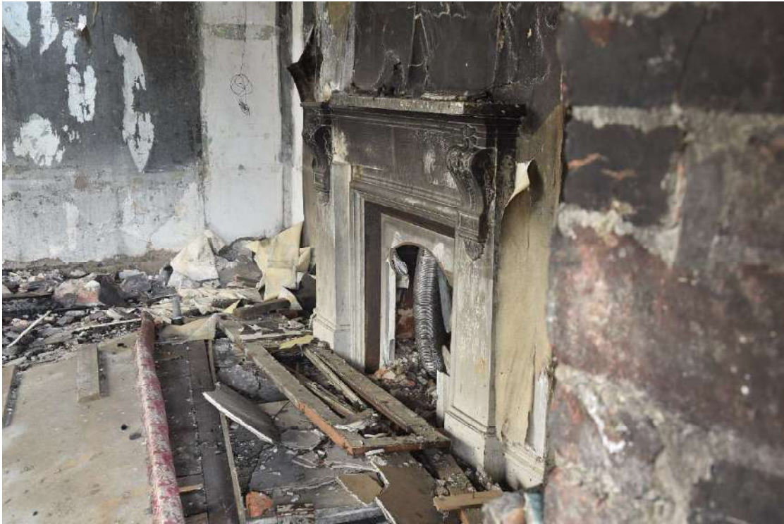
Photo 39: Fireplace in the east wall of Hope House, looking north-east
