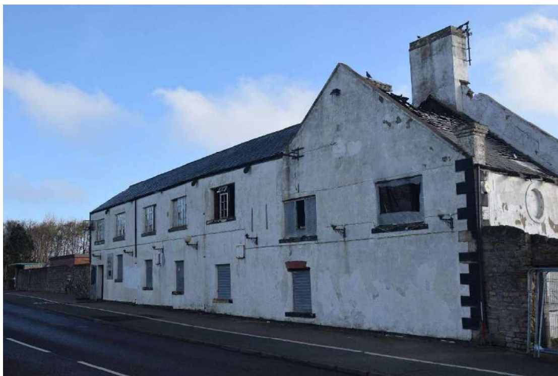
Photo 11: West-facing elevation of Whitburn Lodge with the gable end of the western extension to Hope House visible, looking north-east
