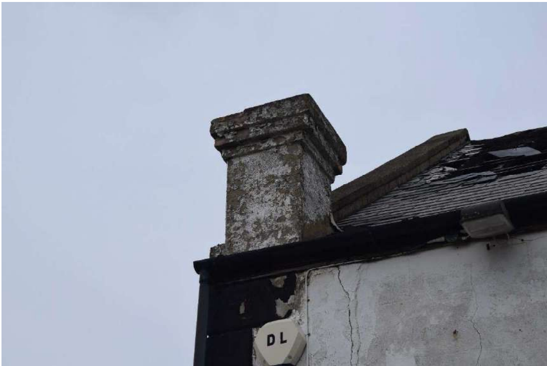
Photo 8: Chimney at the south-west corner of the western extension, looking north
