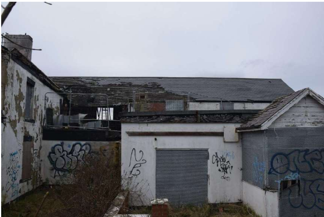
Photo 18: East-facing elevation of the west range, looking west
