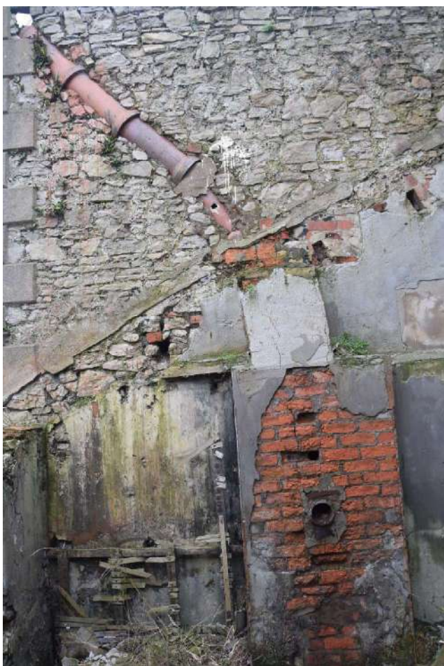
Photo 37 (left): Chimney composed of salt-glazed pipes inserted into the north face of the eastern extension wall of Hope House, looking south
