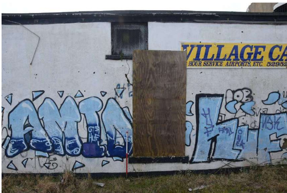
Photo 26 (below): North elevation of eastern horizon showing truncated first floor window, looking south
