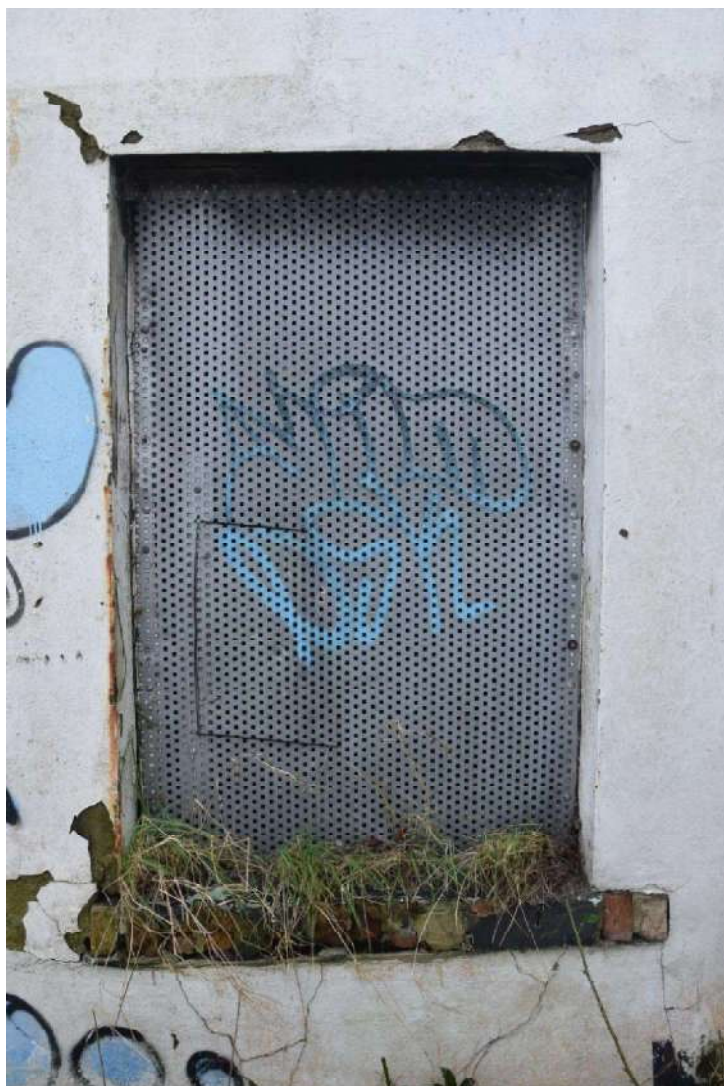
Photo 25 (left): Ground floor window in the eastern extension with a brick sill visible, looking south
