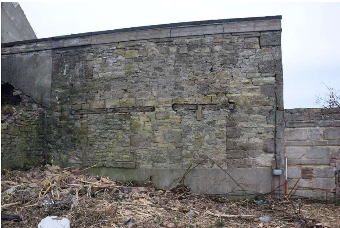
Photo 28: South face of the eastern extension, looking north
