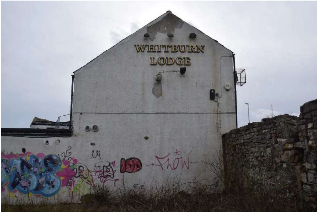
Photo 17: North-facing elevation of the north end of the west range showing the extended length of the east side of the roof, looking south
