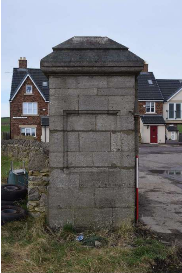
Photo 47: South pier of Whitburn Colliery, looking west
