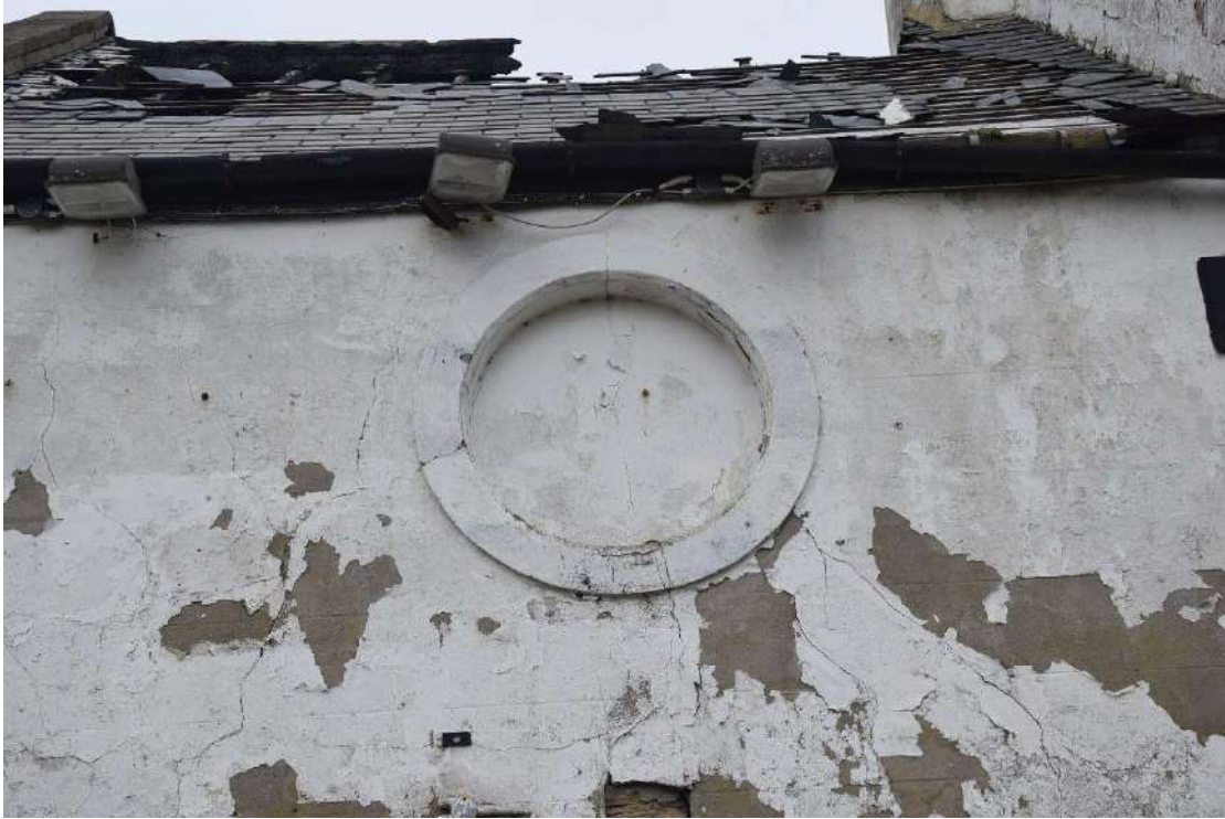
Photo 7: Blank round window in the first floor of the western extension, looking north
