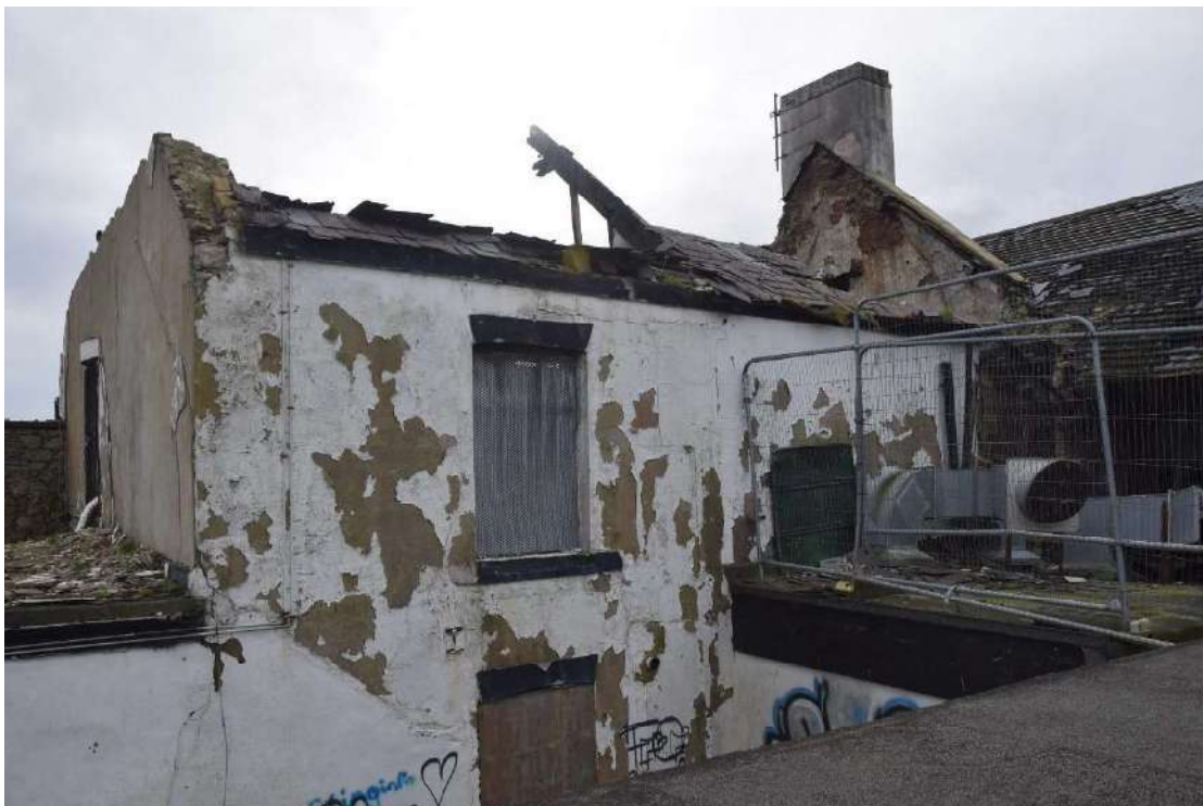
Photo 22 (below): North face of Hope House, looking south-west
