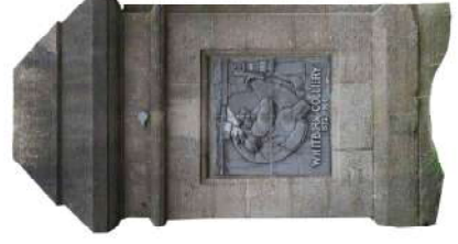
North Pier, west face
