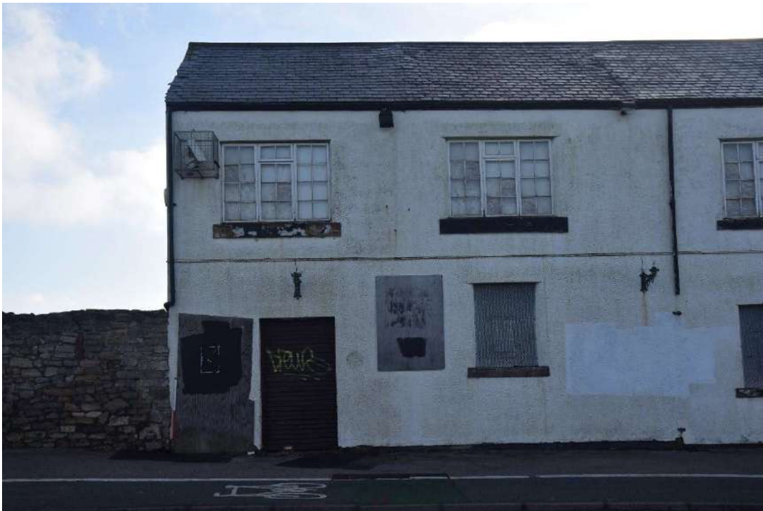
Photo 16: West-facing elevation of the north end of the west range, looking east
