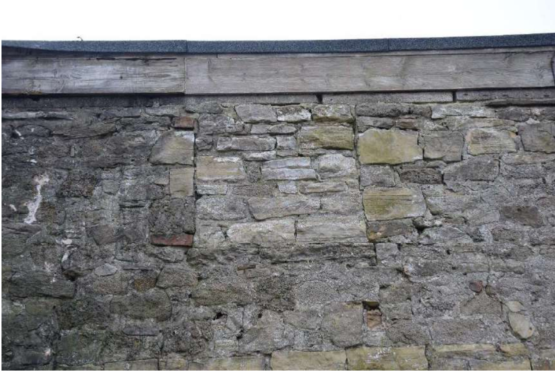
Photo 31: Truncated first-floor window in the south face of the eastern extension, looking north
