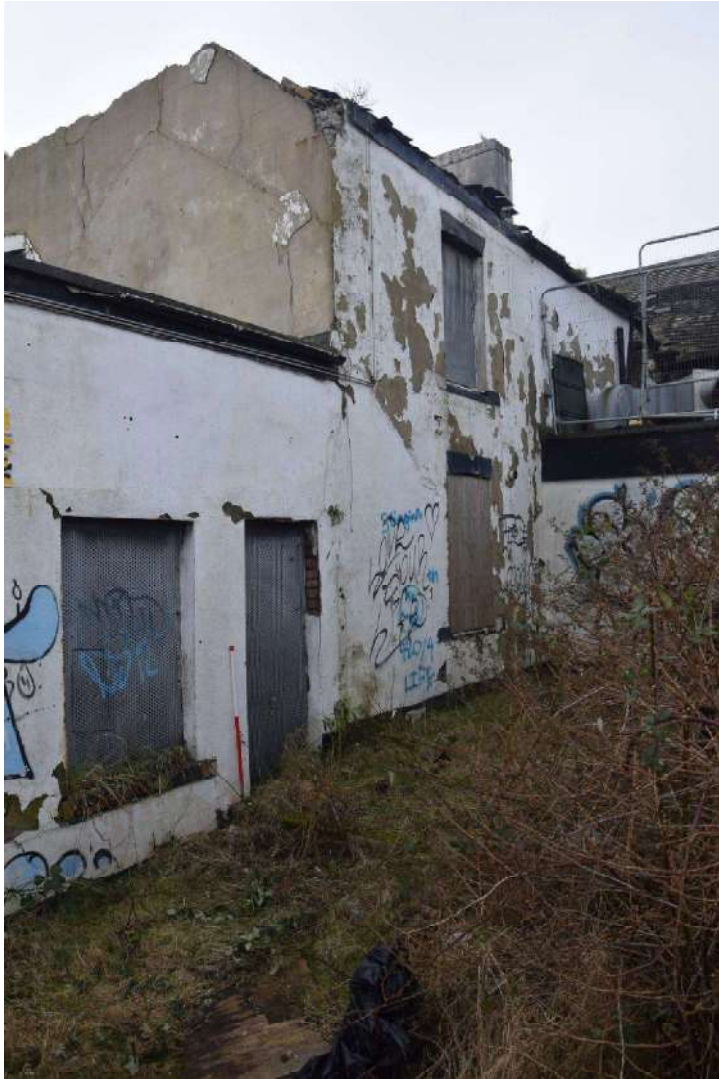
Photo 21 (Left): Oblique view of the north face of Hope House, looking south-west
