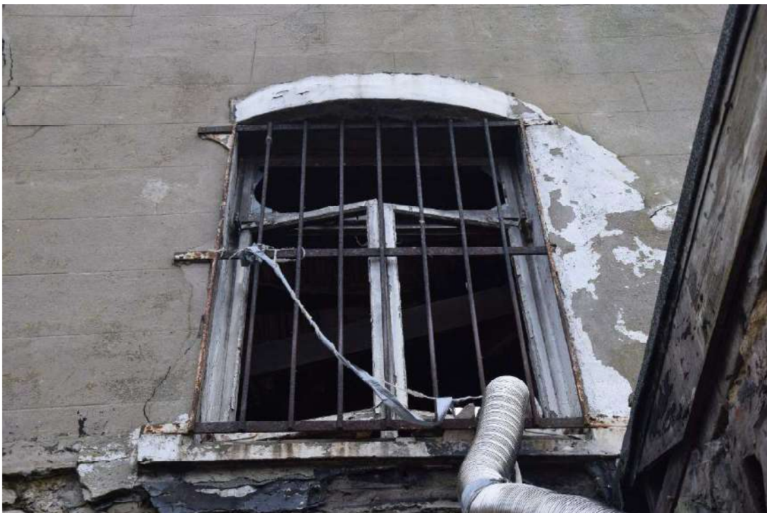
Photo 36: First floor window in the east gable end of Hope House, looking west
