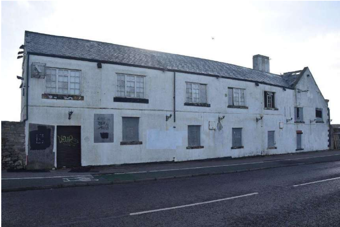
Photo 13: West-facing elevation of Whitburn Lodge showing the cottage which made up the west range of buildings, looking south-east
