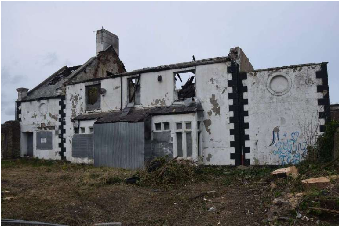
Photo 1: South-facing elevation of Whitburn Lodge showing Hope House, looking north-west
