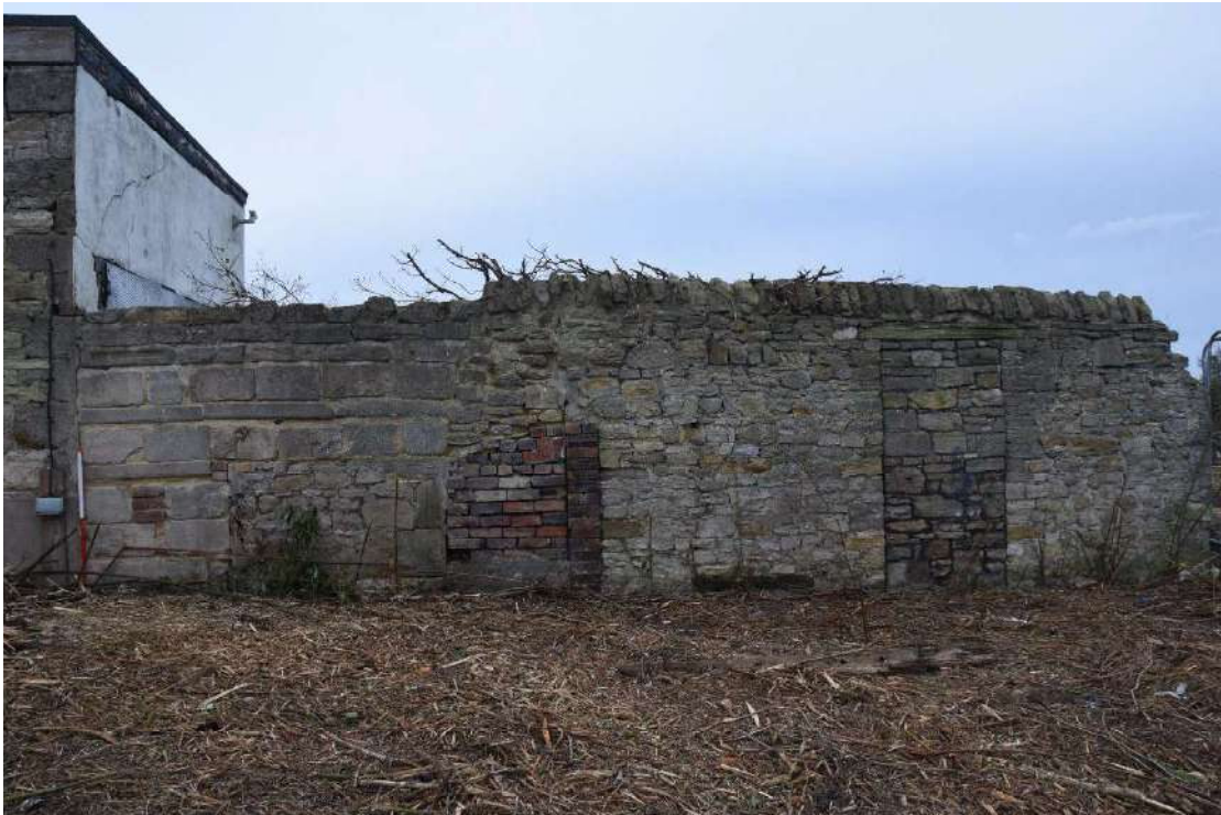
Photo 32: West end of the north garden wall, looking north
