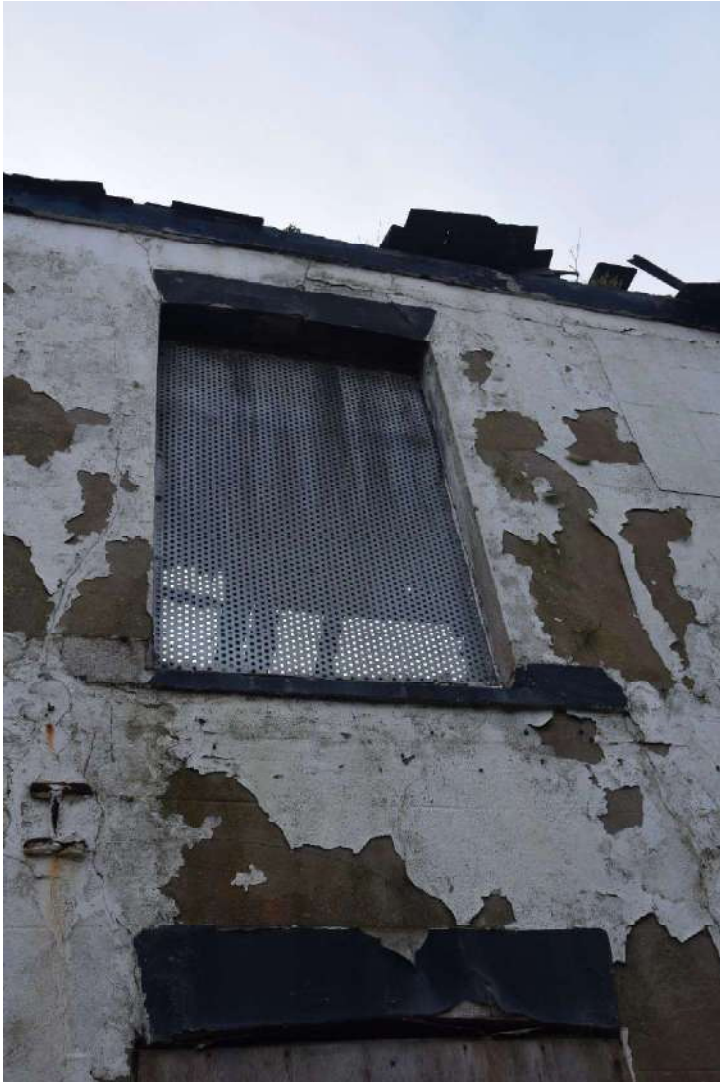
Photo 23 (left): First floor window in the north face of Hope House, looking south
