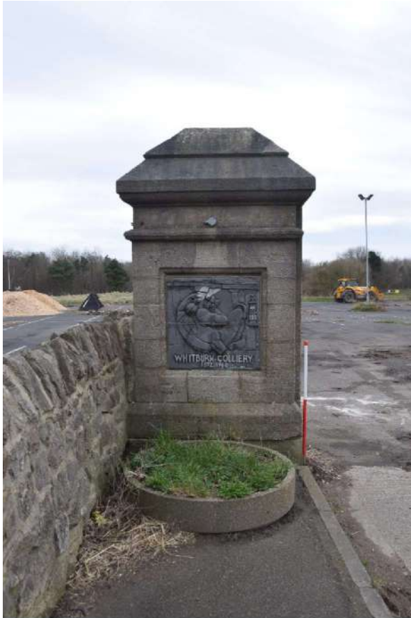
Photo 41: North pier of Whitburn Colliery, looking east
