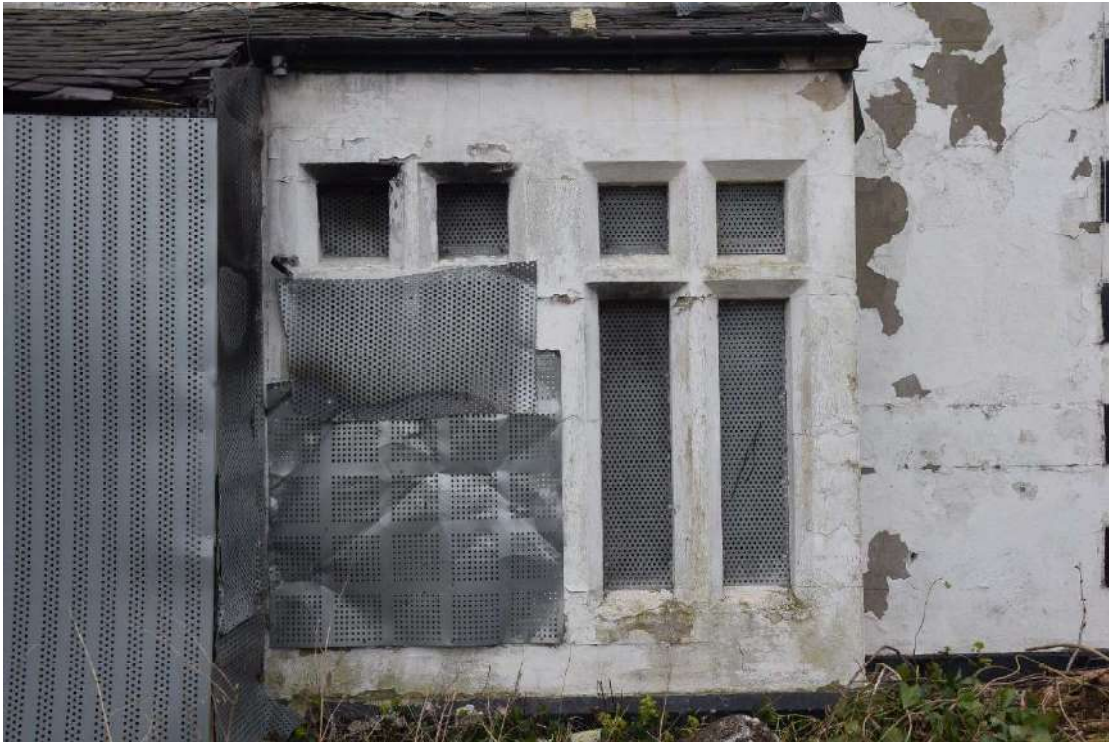
Photo 3: Eastern bay window of Hope House partially obscured by shuttering, looking north
