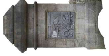
South Pier, west face
