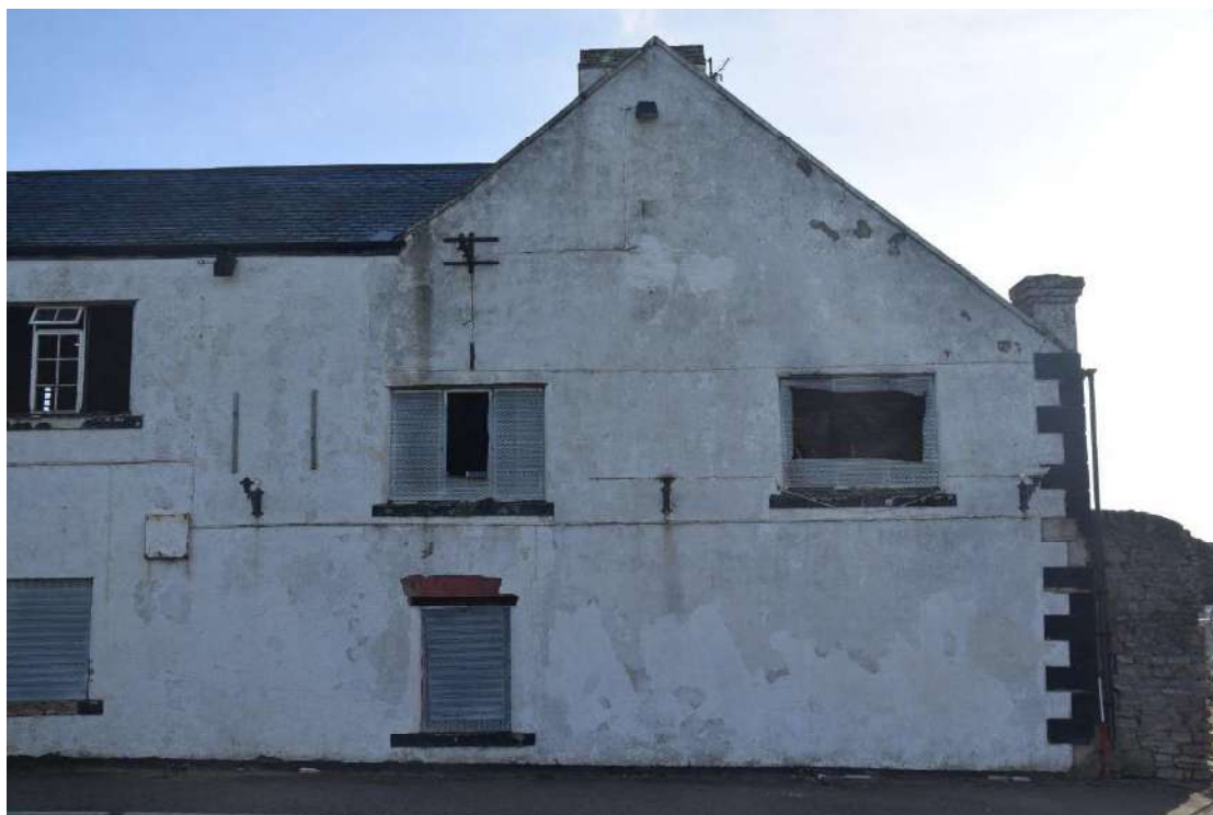
Photo 12: West-facing elevation of the gable end of the extension to Hope House, looking east
