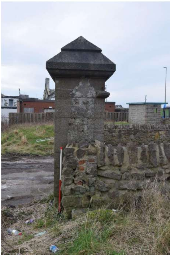
Photo 44: North pier of Whitburn Colliery, looking south
