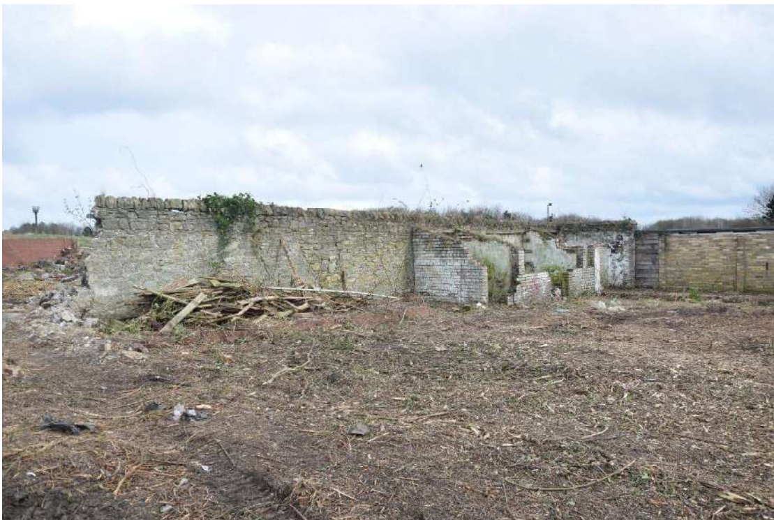
Photo 34: East end of the north garden wall, looking north-east
