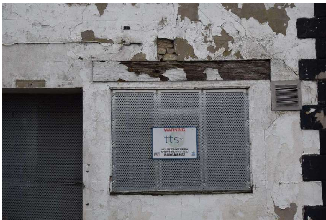
Photo 6 (below): Ground floor window in the western extension to Hope House with wooden lintel above, looking north
