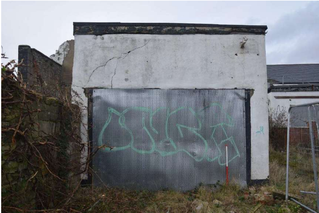
Photo 27: Double-door opening to the eastern extension, looking west
